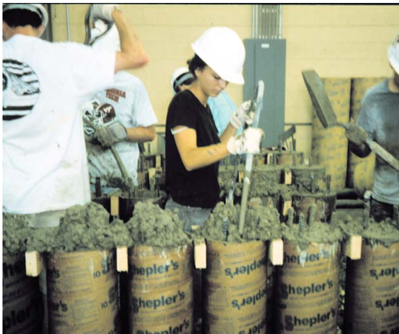
Figure 5.4 Vibrating Concrete in Columns
