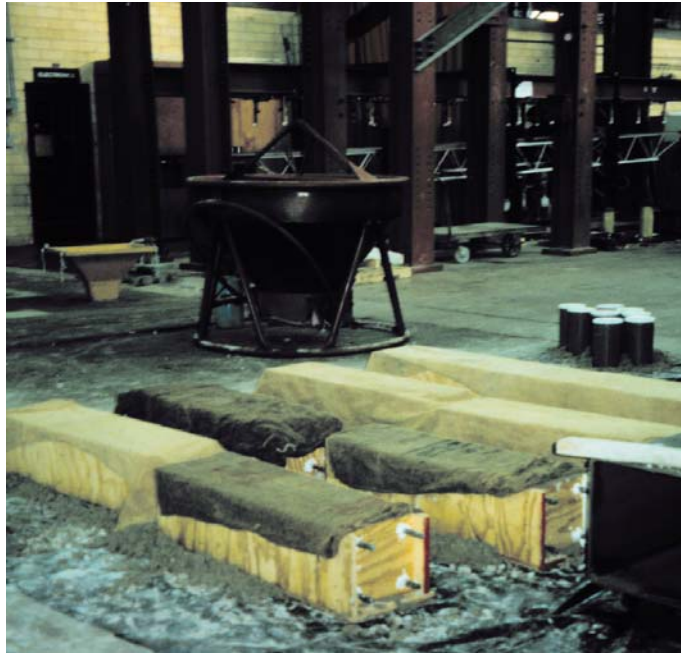
Figure 5.5 Wet-Mat Curing of Beams
