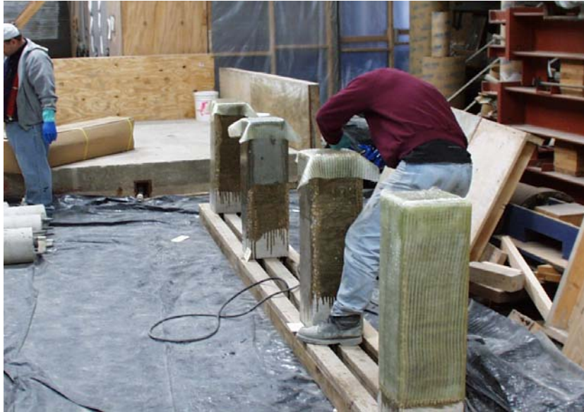
Figure 6.4 Wrapping Beams
