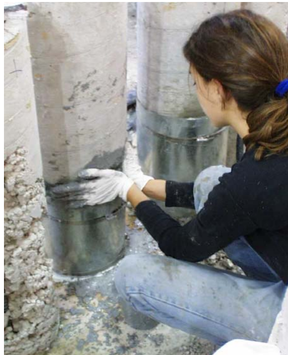
Figure 5.11 Drypacking
