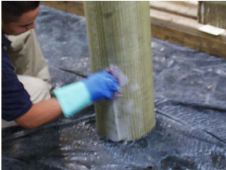
Figure 6.6 Sealing Joints of Column Wrap
