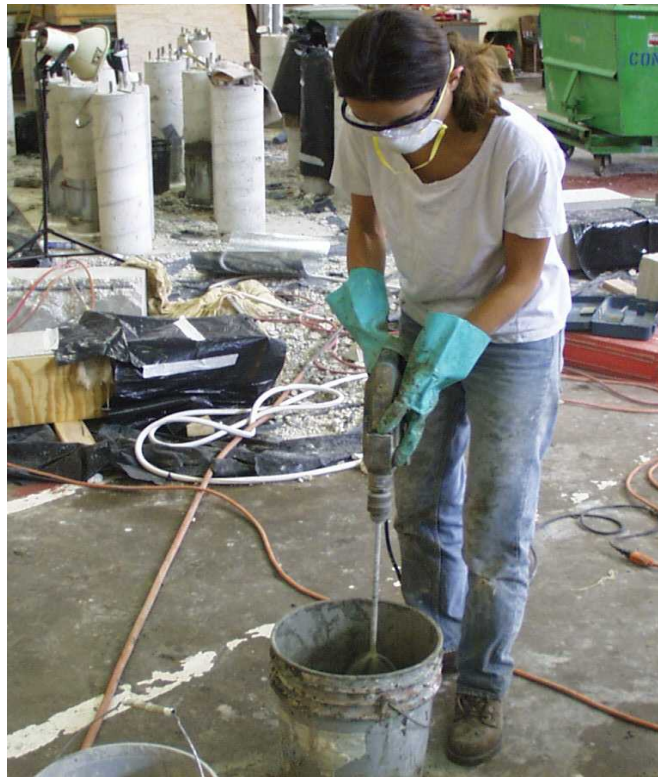
Figure 5.9 Mixing the Repair Materials
