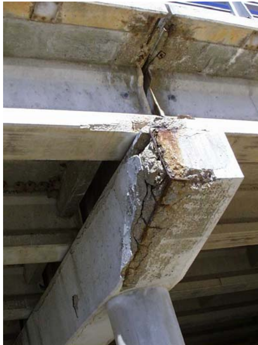
Figure 2.1 Endcap Delamination
