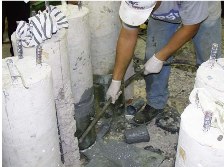
Figure 5.10 Vibrating the Columns
