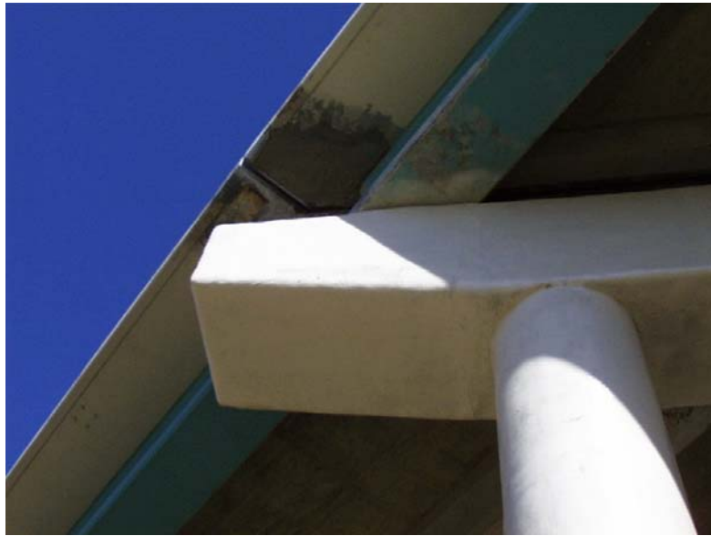
Figure 2.2 Wrapped beam end
