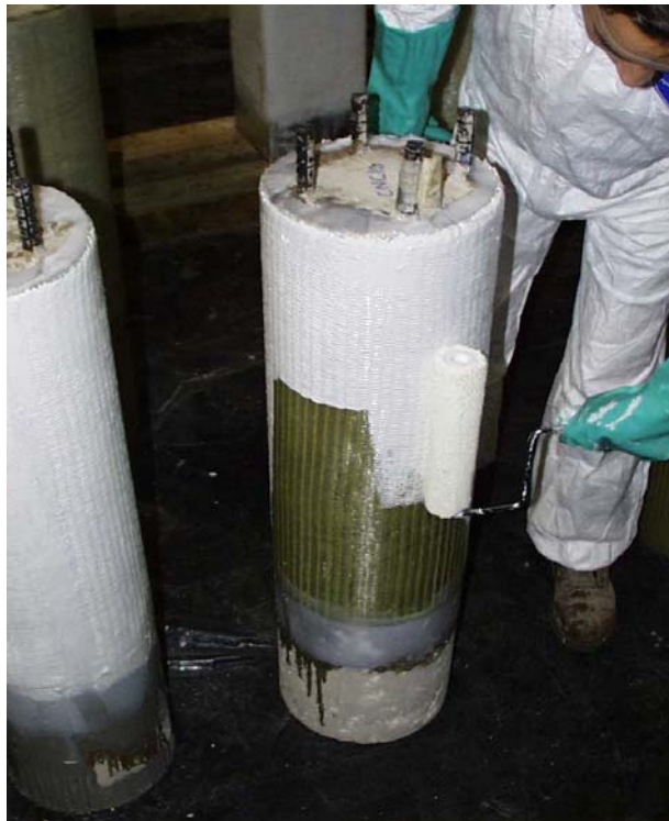
Figure 6.7 Painting Wrapped Column
