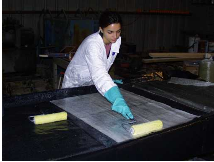
Figure 6.2 Saturating the Fabric with Resin
